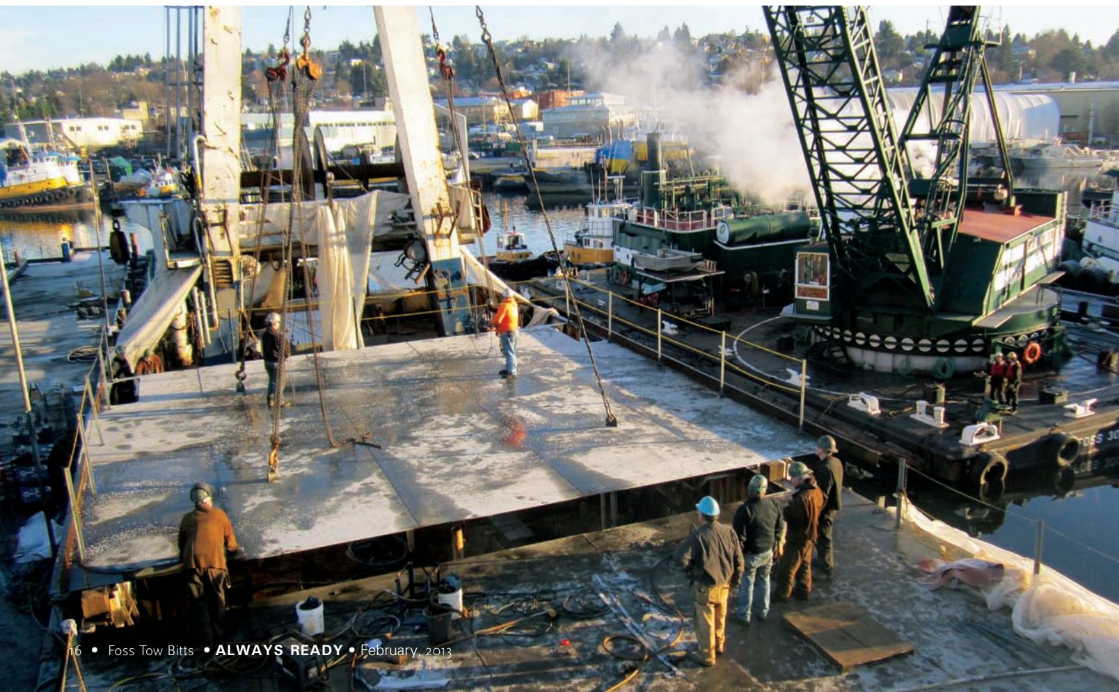
The Foss 300 derrick lowers the second of two prefabricated deck sections into place on the Cape Horn .
